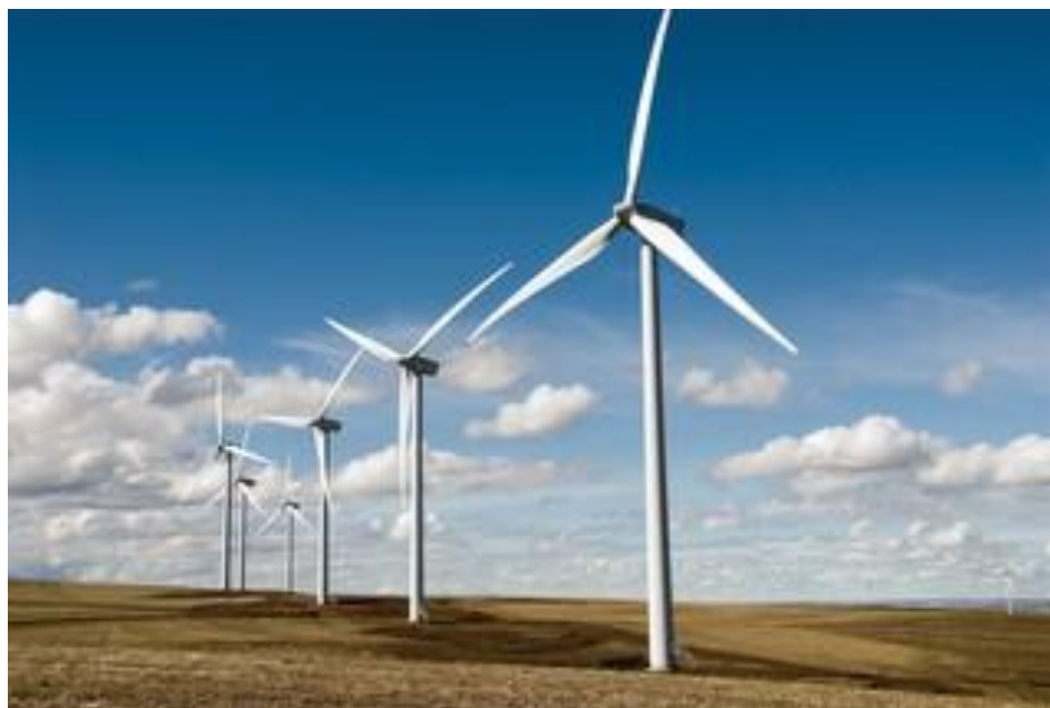
Figure 4-2. Example of a wind farm consisting of horizontal axis wind turbines
