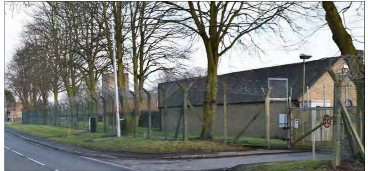
VIEW LOOKING EAST FROM MANTON ROAD TOWARDS PART OF THE OFFICER'S MESS
