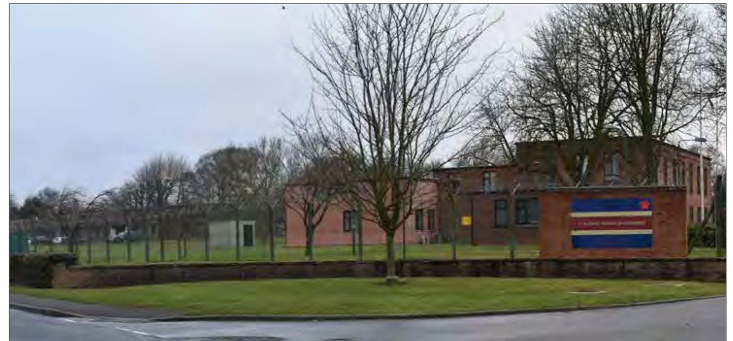
VIEW LOOKING NORTH-EAST FROM EDITH WESTON ROAD TOWARDS PART OF ST GEORGE'S BARRACKS, NEAR THE MAIN ENTRANCE
