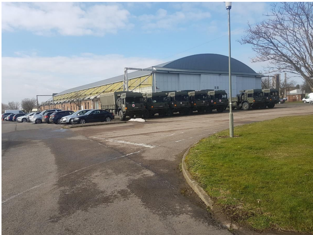
One of the J-Type Hangars on site
