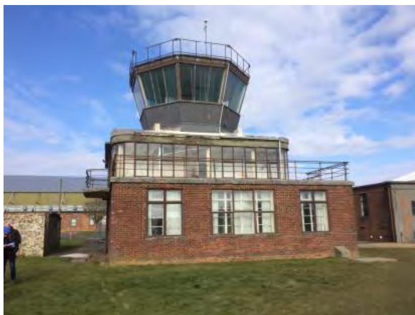
Plate 1: Former Control Tower
