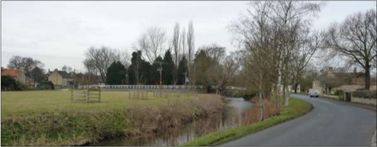
View K from Foundry Road looking west showing Bridge Street across the River Gwash.
