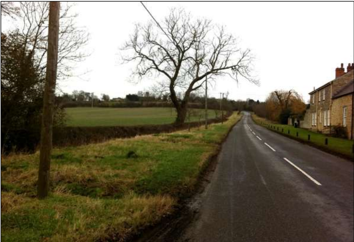
View K; Vista eastwards up and across MO5 to The Old Rectory from Teigh Road, demonstrating the well screened character of Market Overton on the plateau edge.
