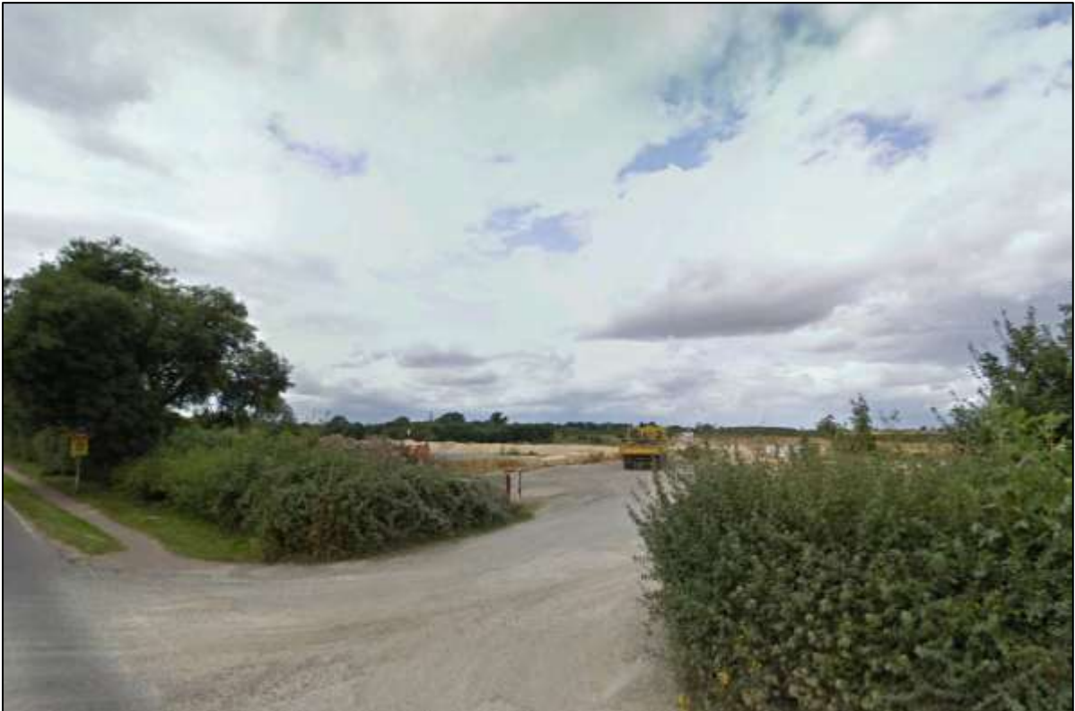
View G from Stretton Road (B668) looking west across G3 at Greetham Quarry.
