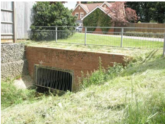
Plate 5.1 a) Schofield Road Culvert and b) Attenuation Basin
