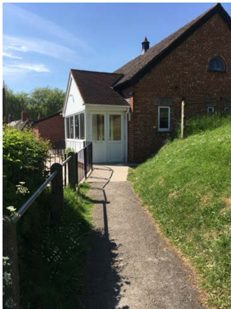
Picture 1 – Path to entrance showing ramp and handrail
