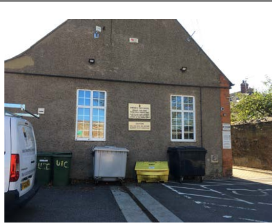
Picture 1 – Approach for wheelchair access 1
