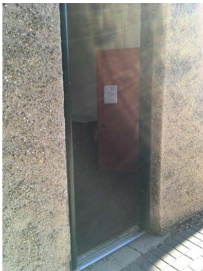
Picture 3 – Approach for wheelchair access 3
