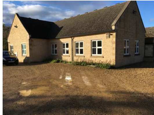
Picture 2 – External picture of building
