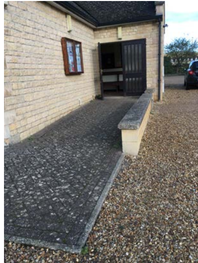
Picture 3 – Approach for wheelchair access from car park
