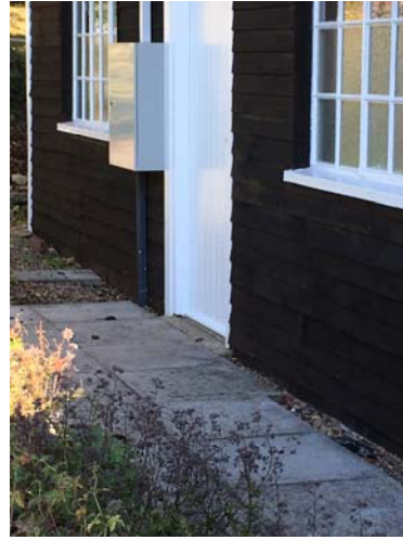
Picture 6 – Level access round side of building
