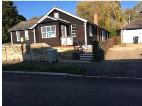
Picture 2 – External view
