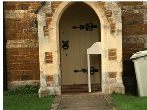
Picture 4 – Wheelchair access door
