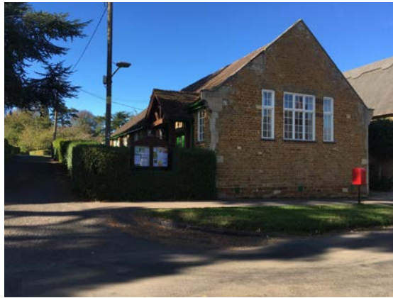
Picture 1 – External view
