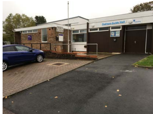
Picture 2 – Access for disabled
