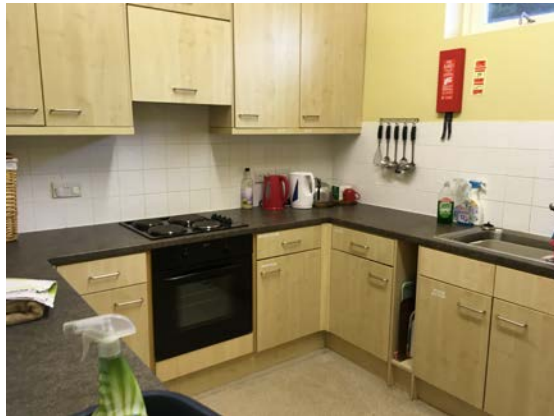
Picture 9 – kitchen facility
