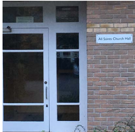
Picture 4 – Front of building signage station
