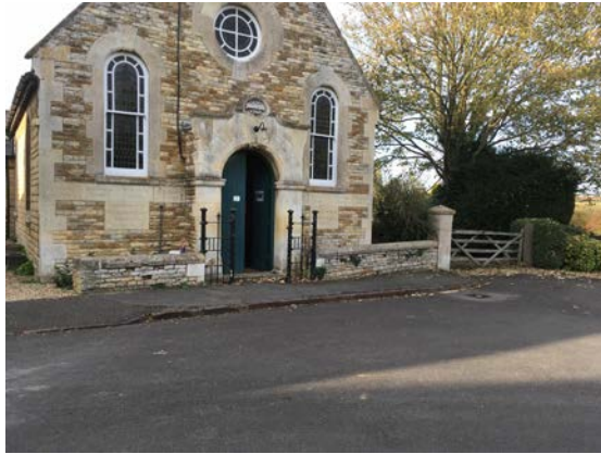
Picture 1 – External view with dropped access
