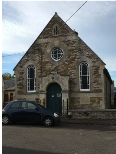
Picture 2 – External view
