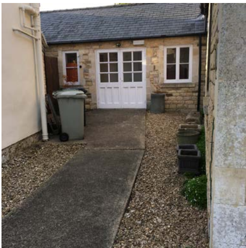
Picture 3 – Wheelchair access
