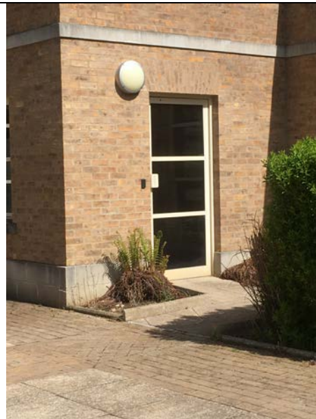
Picture 2 Entrance from Car Park (permanent ramp)
