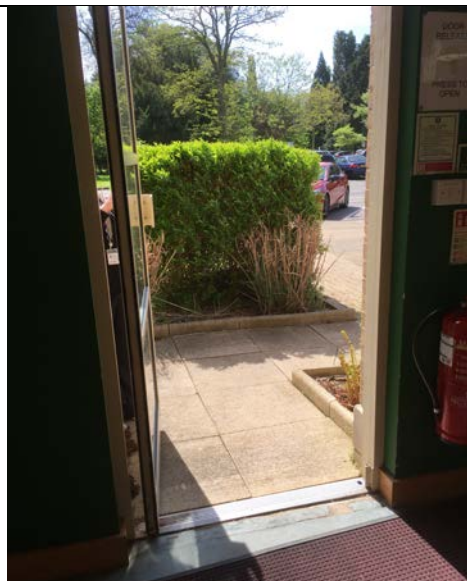
Picture 3 View of ramp from inside entrance
