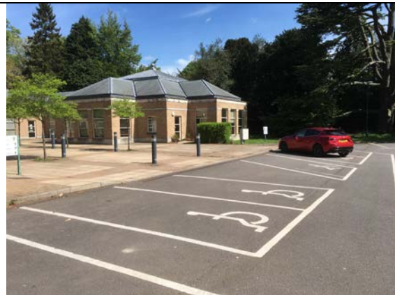
Picture 1 Car Park with disabled parking area
