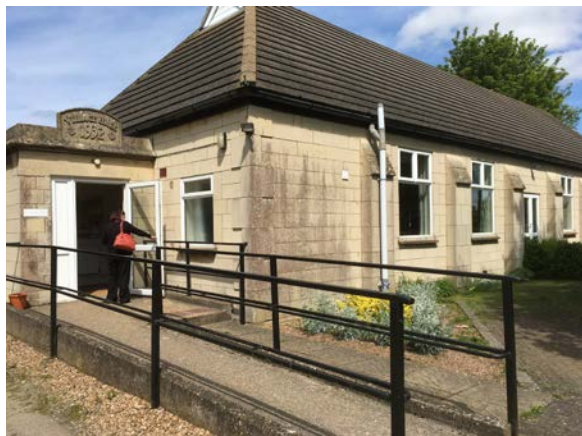
Picture 1 – Entrance showing access ramp and hand rail
