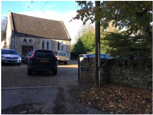
Picture 1 – External view of building/car parking
