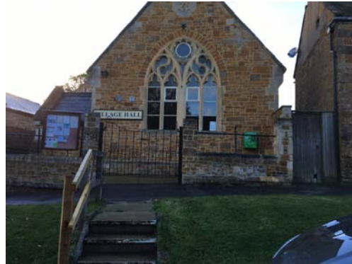
Picture 2 – External View
