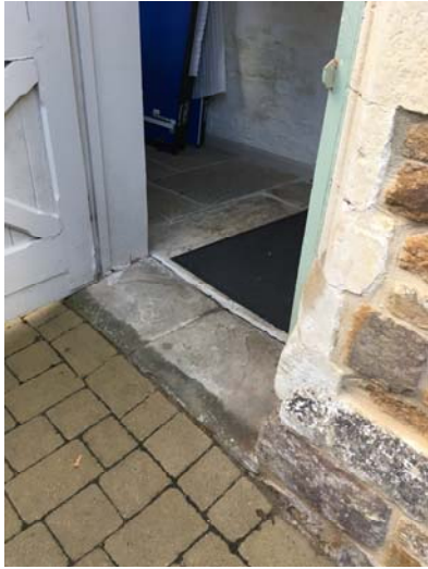
Picture 5 – Level access through main door
