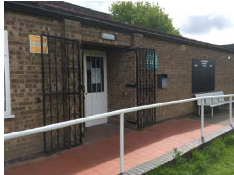
Picture 2 – Entrance showing access ramp and hand rail
