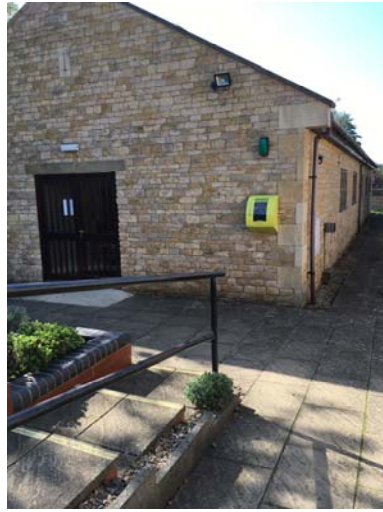
Picture 2 – Front door
