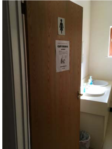
Picture 6 – toilet facilities
