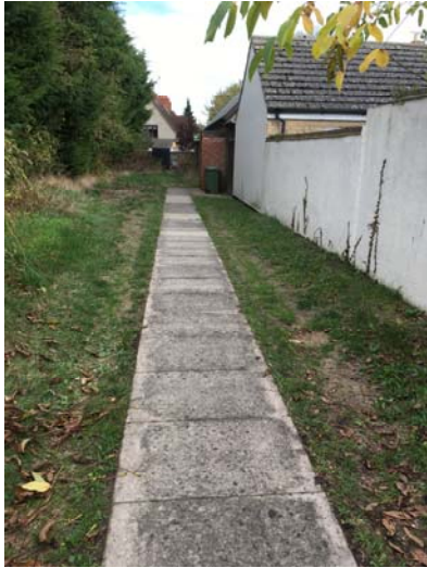
Picture 1 – Path to station
