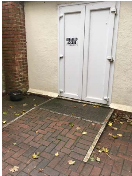
Picture 5 – Access for disabled
