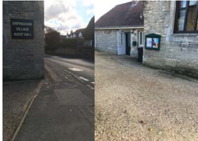
Picture 1 – External view
