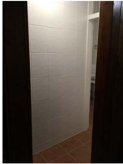
Picture 6 – Toilet facilities
