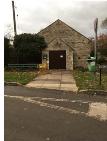
Picture 4 – Level access through main door
