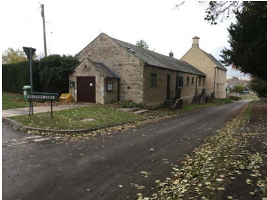
Picture 3 – External View
