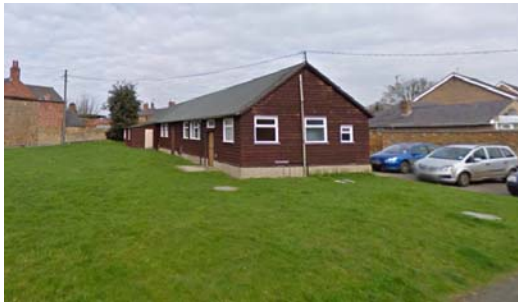
Picture 1 – External view
