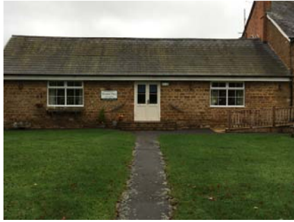
Picture 1 – External view
