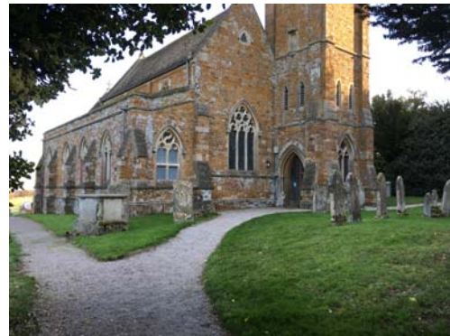
Picture 2 – Level approach from gate to main entrance
