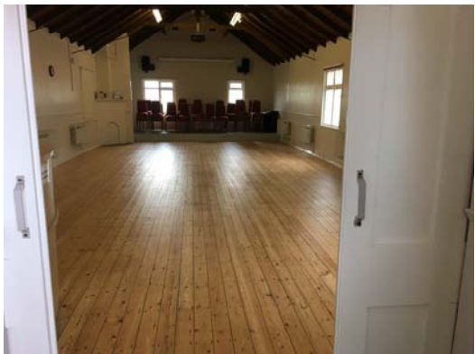
Picture 5 – Main Hall – wooden floor
