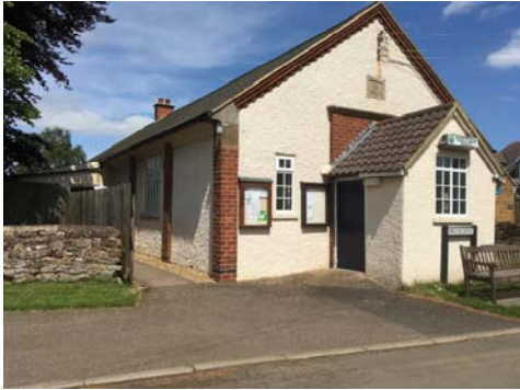
Picture 1 – Entrance showing small access ramp
