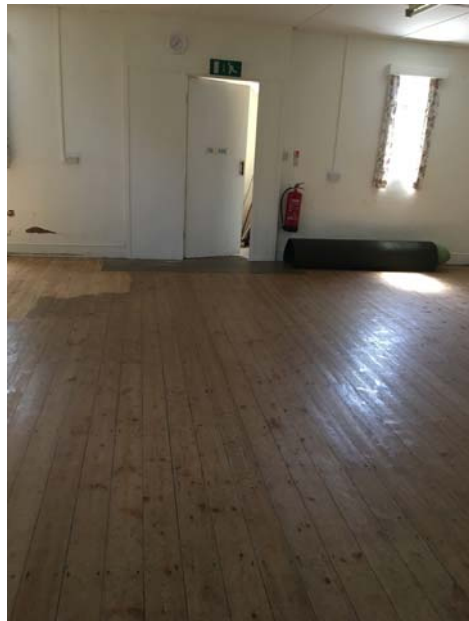
Picture 3 – Polling station area
