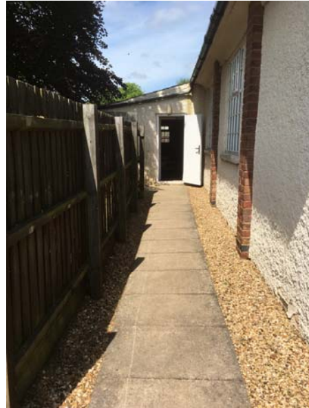
Picture 6 – side entrance to building
