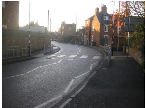
S278 highway contribution for pedestrian crossing North Street West, Uppingham
