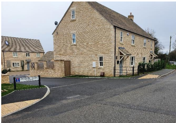
S278 highway contribution for footway construction at Belmesthorpe Lane, Ryhall
